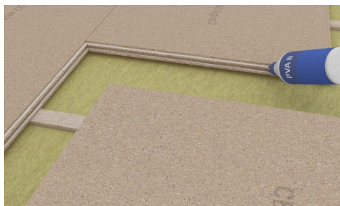
Figure 5 Before assembling the boards, apply plenty of adhesive to both upper sides of the tongue. Remove any glue that is pressed up.
